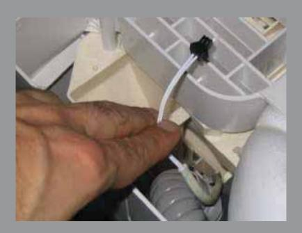
The wiring connection of the defrost wire for the outdoor unit is should be readily accessible through the removable handle. If you cannot find the wire easily, you can locate the connection by removing the top portion of the Outdoor unit. (Please see picture below)
