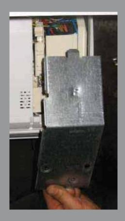
3. Remove the plastic terminal cover. The connection terminals should now be visible.
