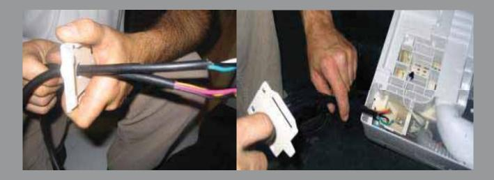
7. Flip the indoor unit over again and pull the wires through the channel.
